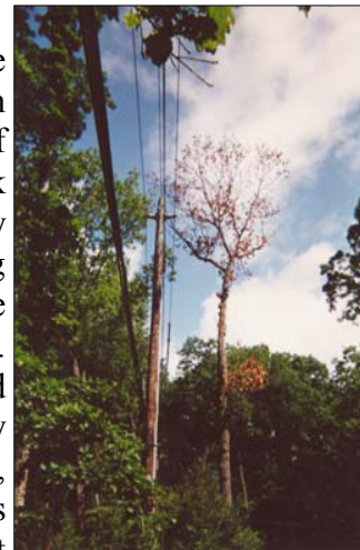
Power line trimming resulted in rapid death of this oak from oak wilt.
