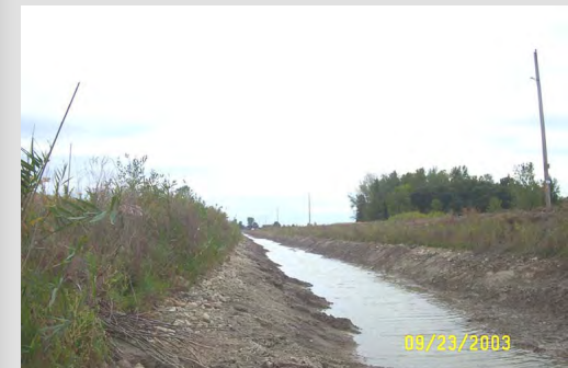
Maintenance of a natural buffer strip between spoils and reconstructed drain prior to drain bank stabilization. Source: Sarah Pistro, Tuscola County Drain Commissioner
