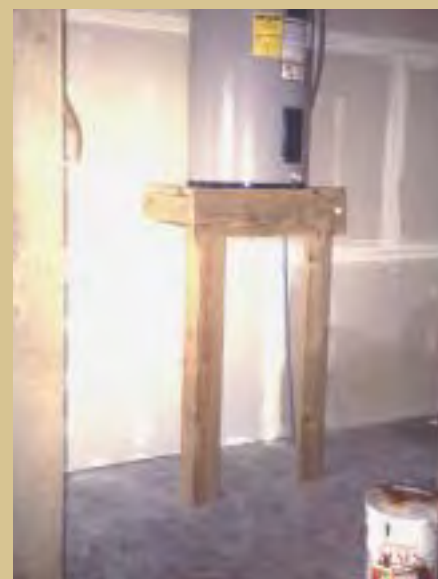
Wet floodproofed garage in Wrightsville Beach, NC.
