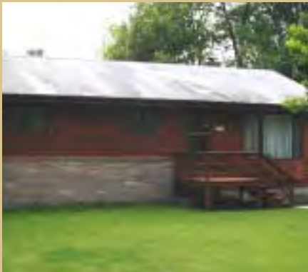
This Illinois home was elevated one foot above the base flood elevation in a shallow floodplain. The site has been flooded several times since the project was completed, but water did not damage the home.
