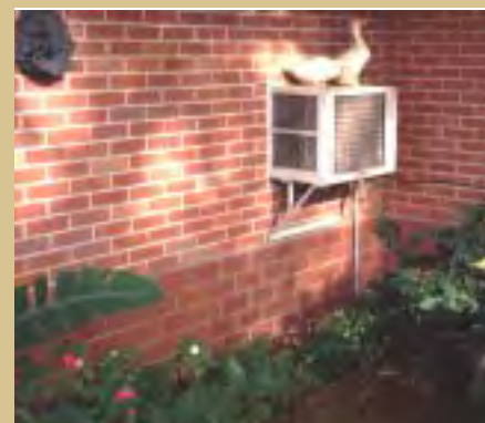
In this dry floodproofed Louisiana house, plastic sheeting is covered by thin facing brick. The building's walls become a watertight barrier to shallow flood waters.
