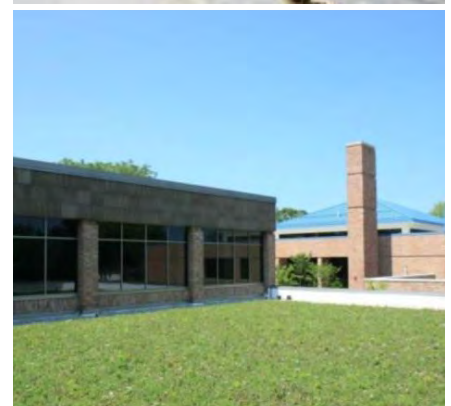
The roof of the Community Center before (top) and after (bottom) a green roof was installed. Source: The City of Grand Haven
